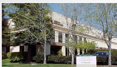
Industrial - 87,500± SF Leased 21062 Forbes Avenue, Hayward INDUSPAC CALIFORNIA, INC.
