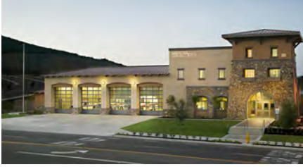
City of San Marcos Fire Station No. 4 on San Elijo Road.
