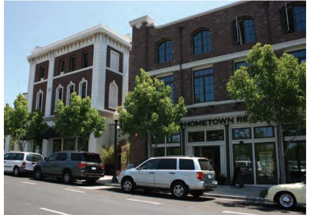
Image 20.225-1 Form-Based Regulation Regulating building form, frontage types, and parking locations focus development of character instead of strictly land use.
