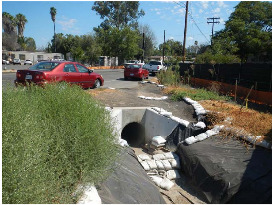
Photo #5: Storm water outlet discharge to site at northwest property corner.
