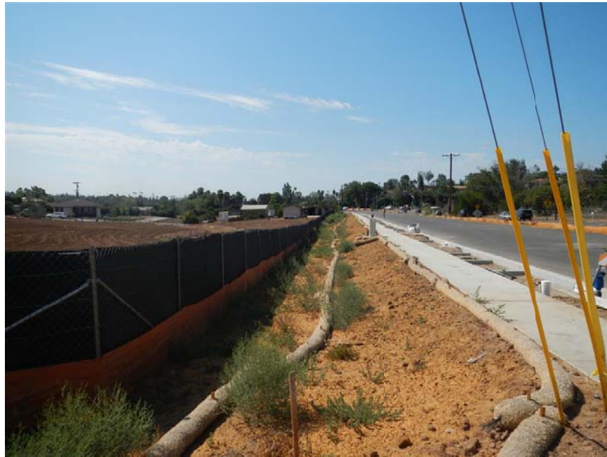
Photo #3: View to south from northwest corner of site; subject property on left and Bear Valley Parkway is on right
