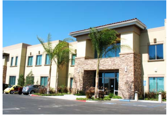
Office complex in Rancho San Diego
