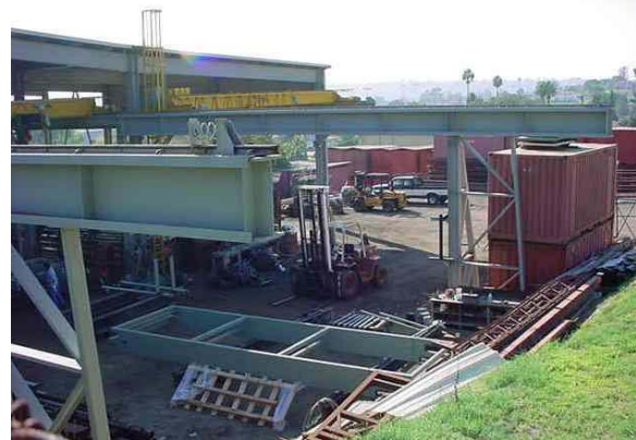
Steel fabricating plant in Spring Valley
