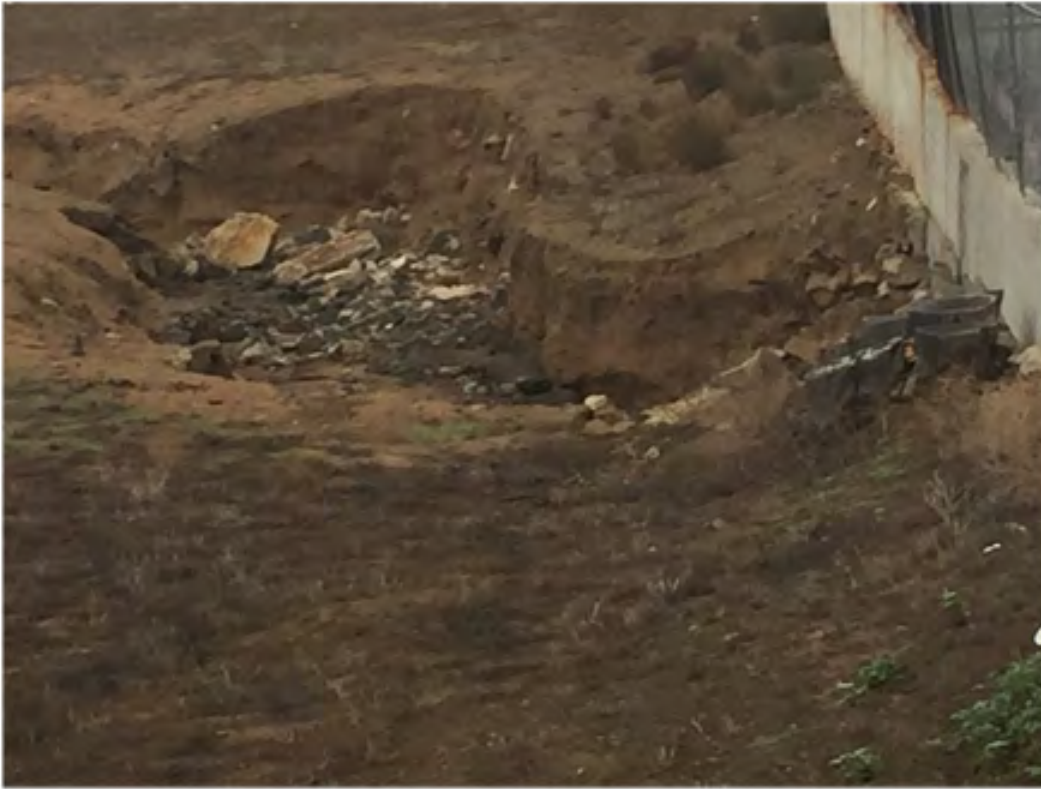
337 East Carmel southeast corner facing north
