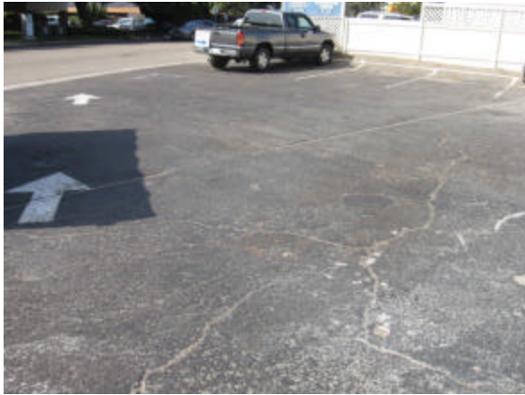
Photo #27 Driveway and parking area of 343 South Highway 101 – southwesterly view.
