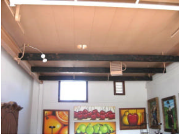
Photo #25 Interior of former gas station building, recently renovated with new drywall and paint.
