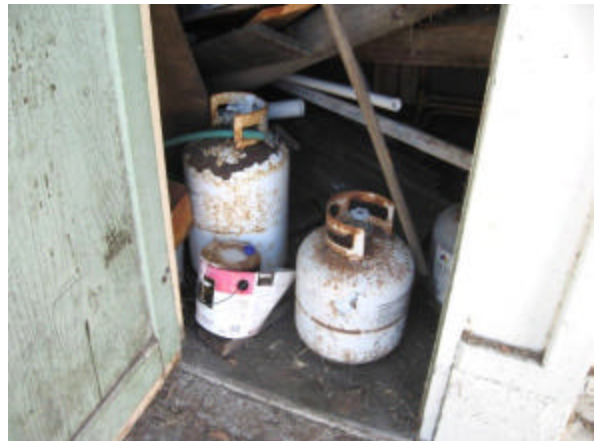
Photo #34 Storage room within the ombudsman building containing small amounts of paint and empty propane gas cylinders.
