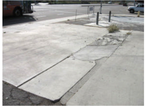
Photo #26 Alternate view of former gas station fuel pump islands (two).
