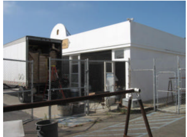
Photo #22 Southwest view of former gas station.
