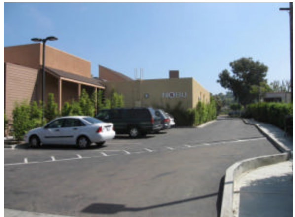
Photo #12 Alternate view of north adjoining property – easterly view.
