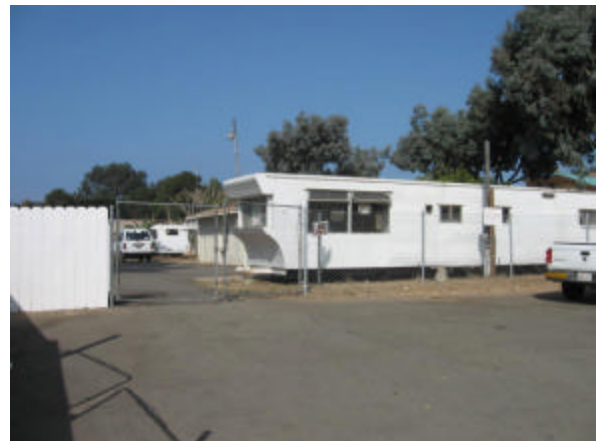
Photo #18 East entrance into trailer park, 329 South Highway 101.
