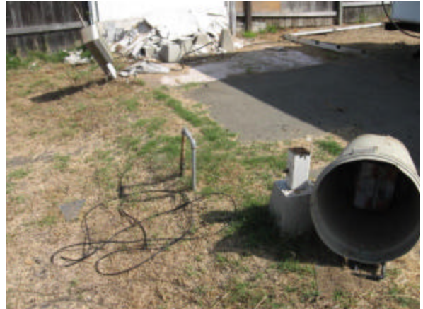
Photo #32 North central portion of trailer park showing typical gas and power hook-ups. Construction debris pile shown in background.
