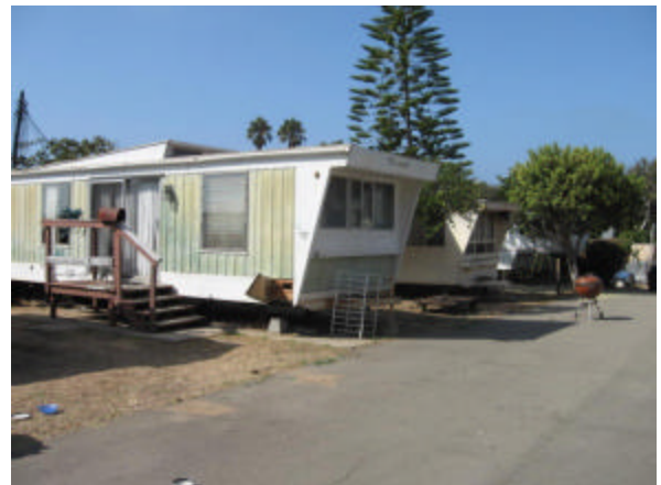
Photo #30 Vacated trailers and driveway of trailer park – southwesterly view.
