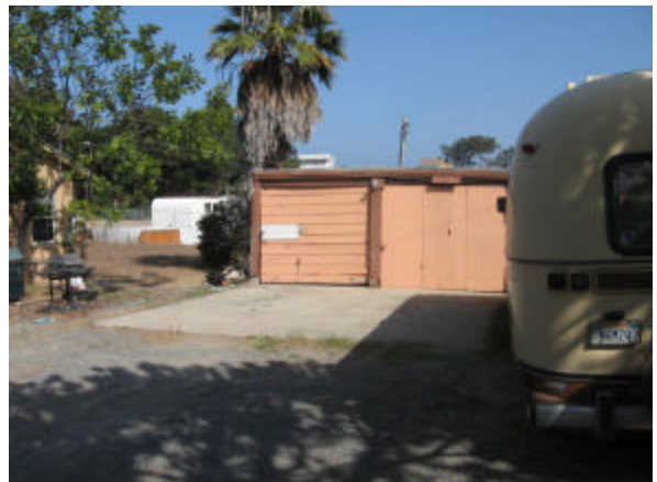
Photo #6 Wood and metal storage shed at 128 Dahlia Drive – northerly view.
