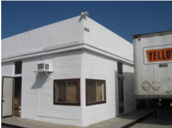
Photo #21 Northwest view of former gas station building at 343 South Highway 101. The building is currently used as a furniture/antique store.
