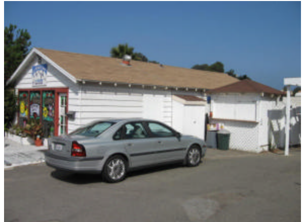
Photo #4 Hair salon located at 120 Dahlia Drive, south side of site – northwesterly view.
