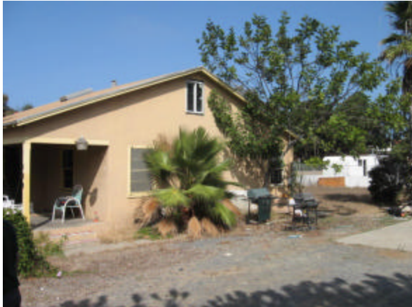
Photo #7 Vacated house at 128 Dahlia Drive – northwesterly view.
