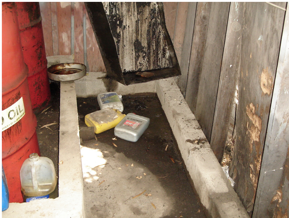
Photograph #9 View of oily stain on concrete floor in shed containing waste oil and waste anti-freeze at Uruapan Auto Dismantling.
