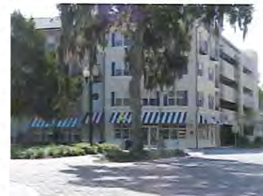
Ground level retail shops are part of parking structure designs.
