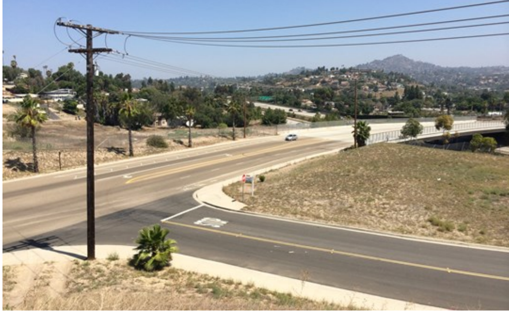
7. Looking north-northeast from northeast portion of property.
