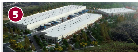
Pacific Vista Commerce Center Class A 5-Star Industrial Warehouse
