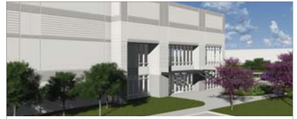
424,280 SF 2800 S. Millers Ferry Rd. Wilmer, TX
