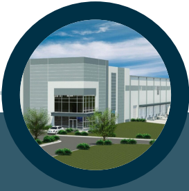
381 DAVIS LAKE RD GARDNER LOGISTICS PARK - PHASE III
