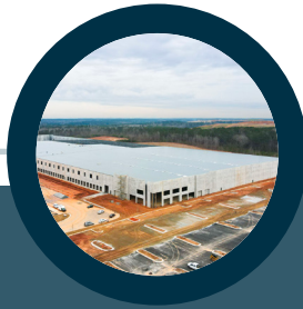
700 PALMETTO LOGISTICS PKY - BLD 3 PALMETTO LOGISTICS PARK
