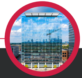
201 17TH STREET NW ATLANTIC STATION
