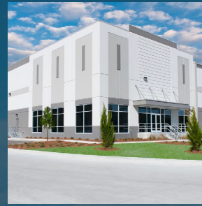
2509 DEAN FOREST RD. | BLDG. A SAVANNAH, GA 31408
