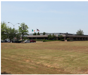
14117 INDUSTRIAL PARK BLVD NE COVINGTON, GA 30014
