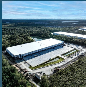
NORTHGATE INDUSTRIAL - BLDG. 3 RINCON, GA 31326
