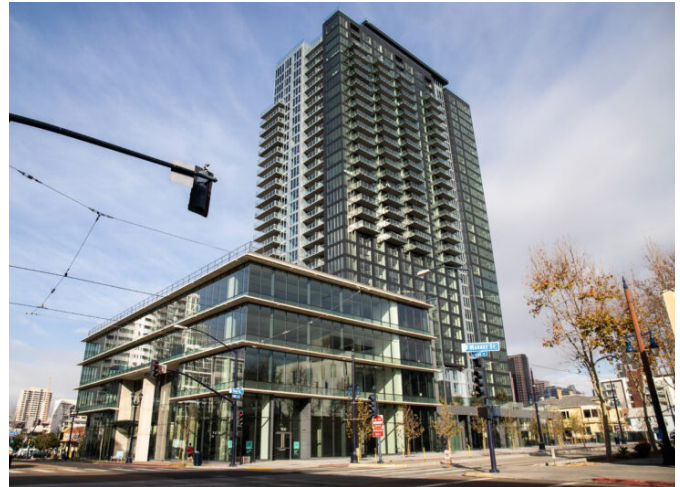
A mixed-use downtown project by Holland Partners includes a UCSD satellite and rental housing. Published by Voice of San Diego.
