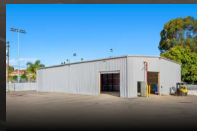
±4,700 SF METAL BUILDING
