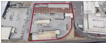
80,000 SF 800 77th Avenue Oakland, CA
